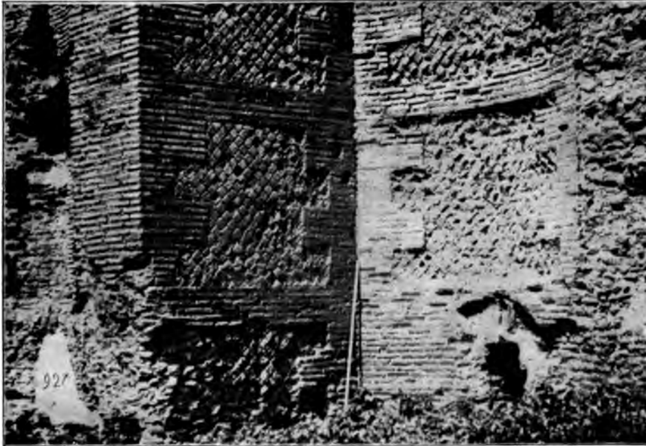
SPECIMEN OF OPUS RETICULATUM , WITH BRICK QUOINS AND "LEVELLERS," AND CONCRETE BODY.
